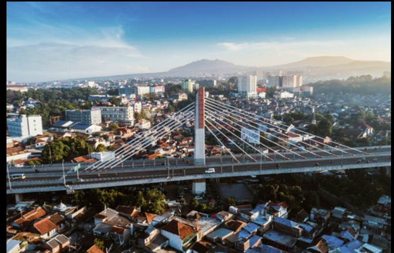
Aerial view of Pasupati Bridge, Bandung
